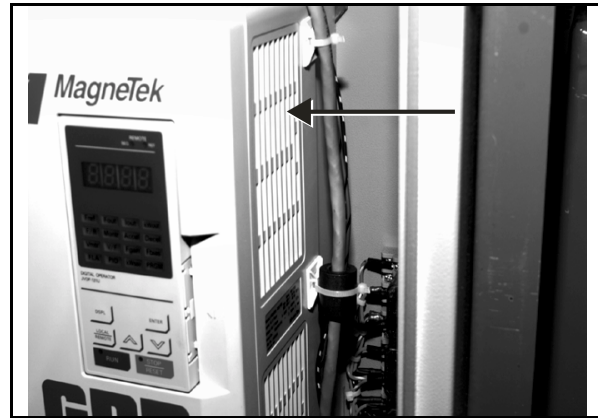
Figure 9: Inverter Vents
